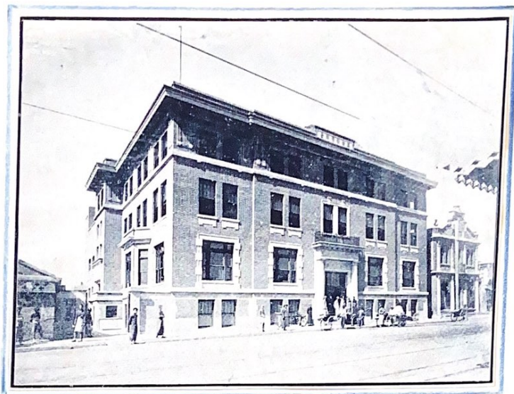
CENTRAL BRANCH - TUNG MALU ACQUIRED IN 1910. 2\frac{1}{2} MU. 112' \times 130' BUILDING ERECTED IN 1914. $114000.00
