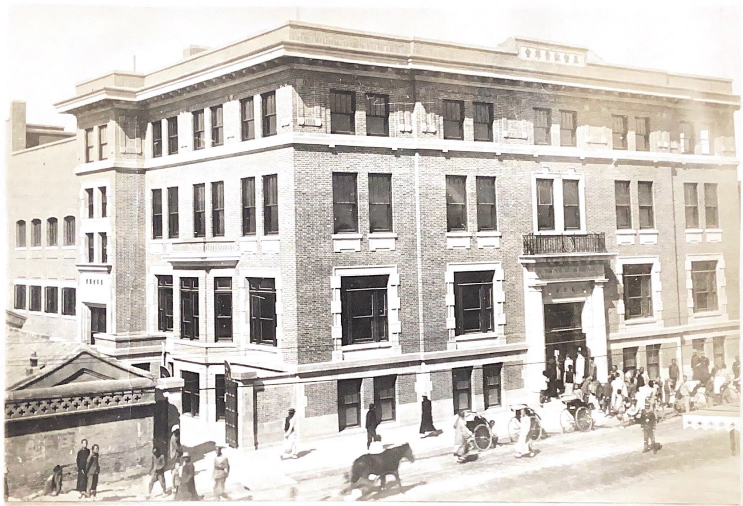
Association Building Tientsin, China
