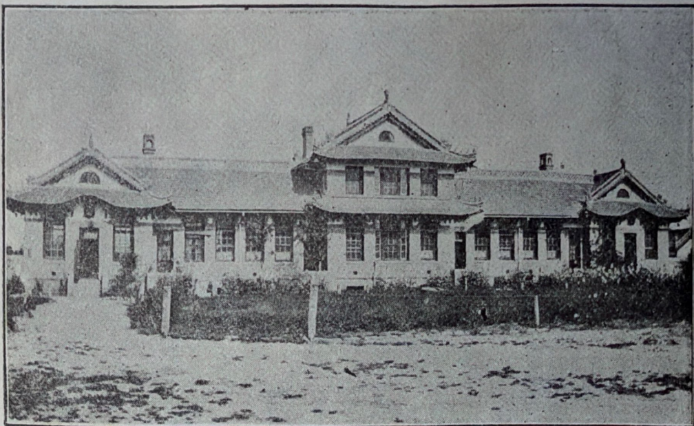
面正院醫美華 Central Building, Linking Memorial Hospital, containing outpatient department, drugroom, offices and operating room.
